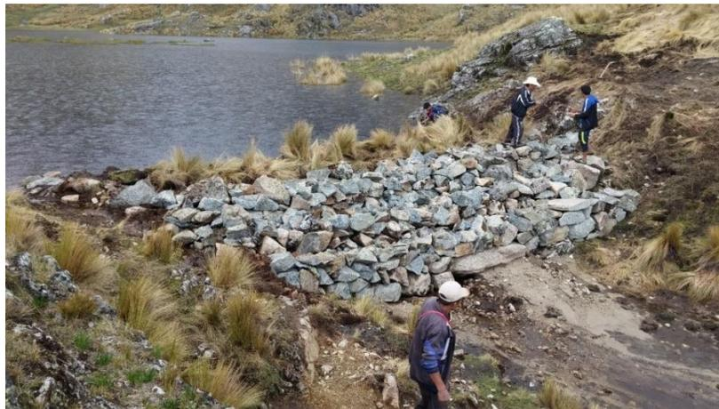
Figure 28 Communal small-scale dam construction in the Mariño watershed. *Source: Ruderson Rivera*
